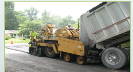
Typical hot mix asphalt paving operation
