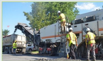
Typical milling operation
